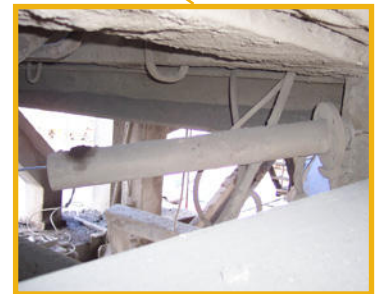
Temperature measurement at mixture discharge chute
