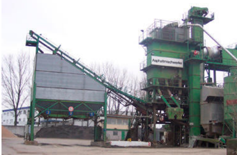
Temperature-controlled asphalt mixing plant
